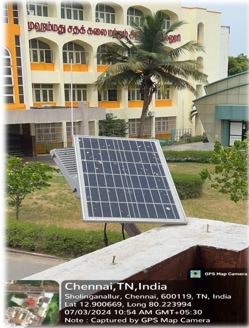
Solar Plant - 1@ Main Building
