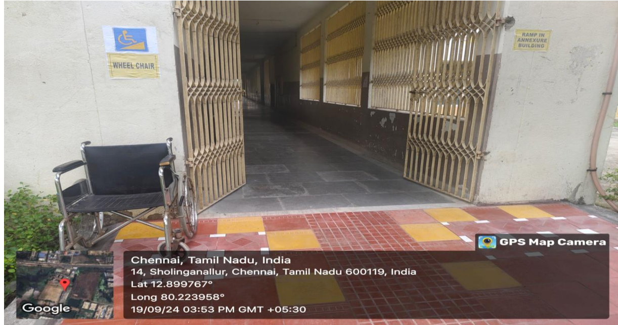
Ramp @ Annexure Main Building
