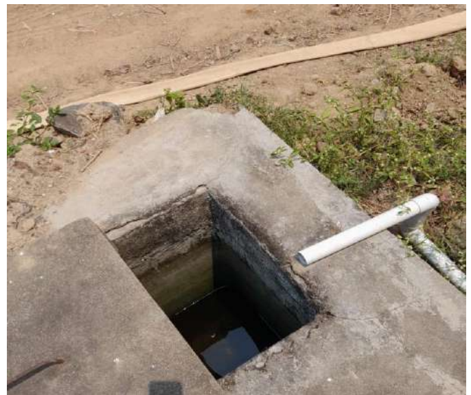
Rain water harvesting percolation pit
